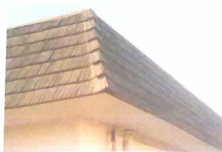
Fig.3. Imitation Roofing Shakes of embossed and painted CBPB (Van elten, 2006).
