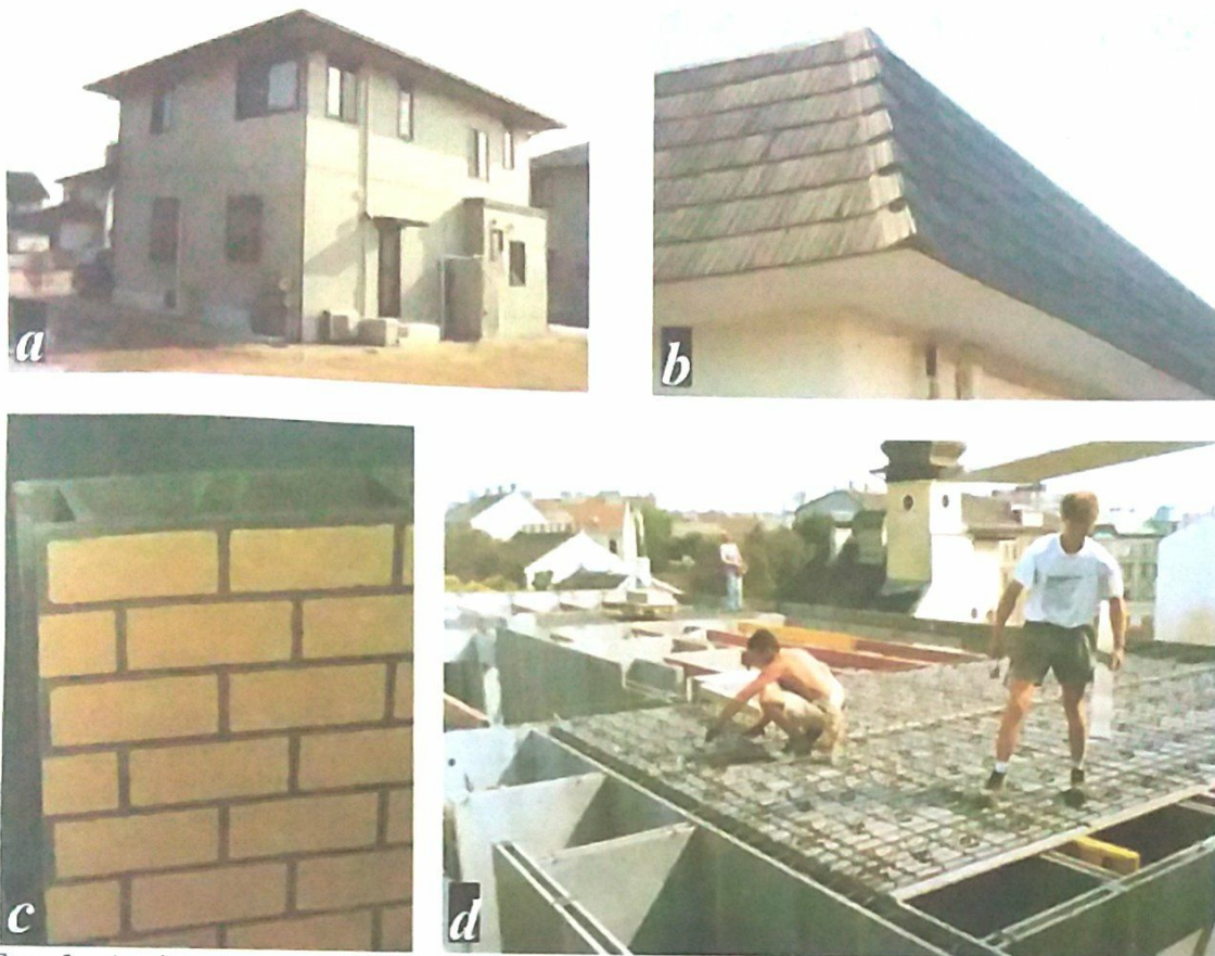
Fig. 2. Applications of CBPB (a) Embossed and painted CBPB for wall claddings, (b) Imitation Roofing Shakes of embossed and painted CBPB, (c) CBPB hollow wall panel, (d) Installation of the CBPB prefabricated floor units
