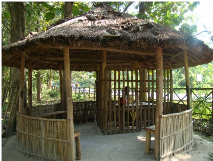
Figure 2.6 The ticket counter
