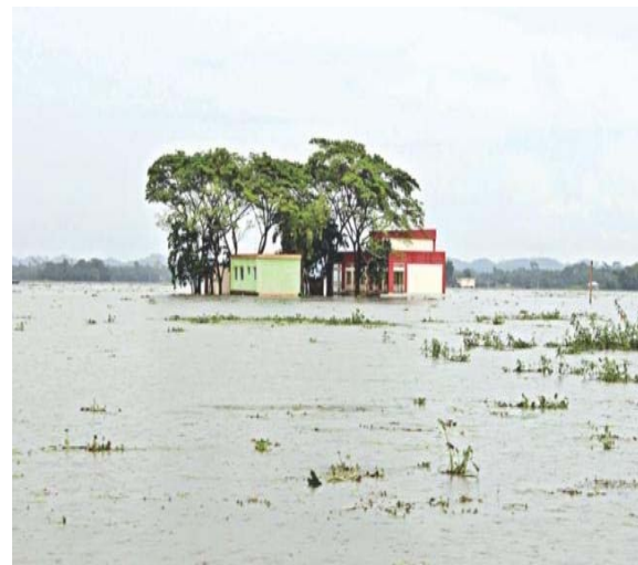
Figure 102: The Kairchak Govt. Primary School in KulauraUpazila of Moulvibazar surrounded by flood water (Source: Star file photo, the Daily Star, 02 July 2017)
