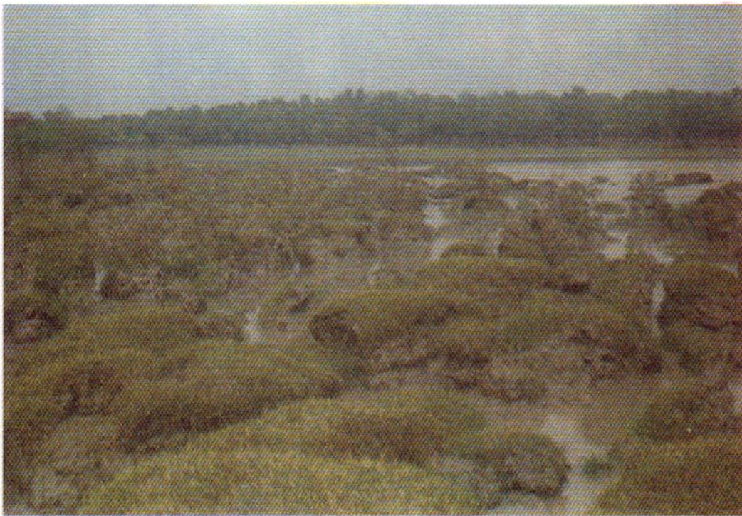
Fig.15h Erosion due to wave and tidal actions
